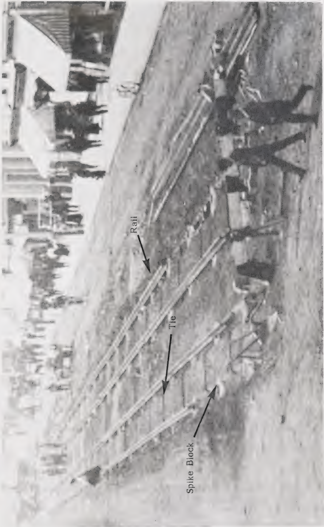
Plate 2. (City of Edmonton Archives) First Stages of Permanent Construction on Jasper Avenue, 1908
